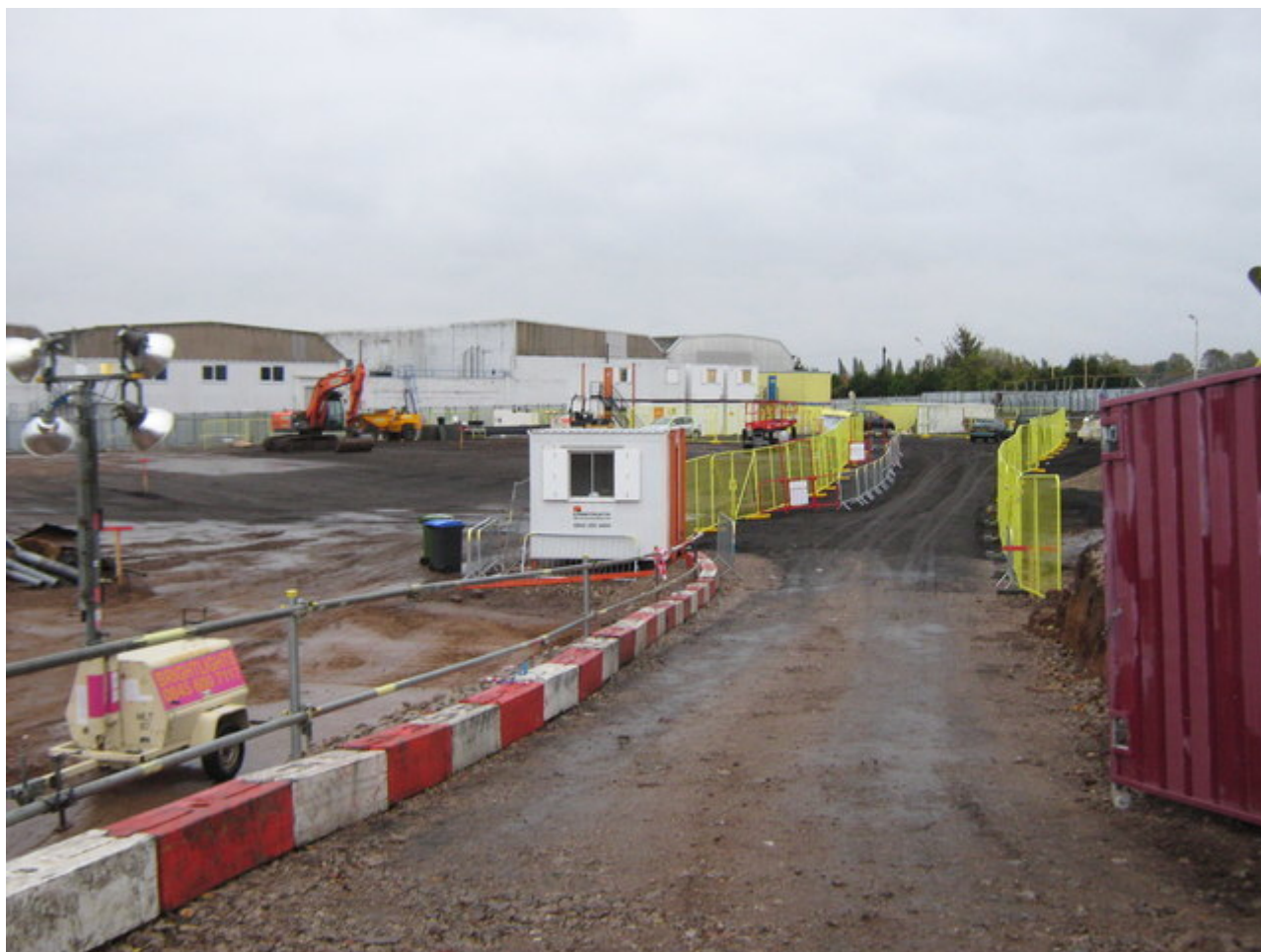
Site access at smith street
